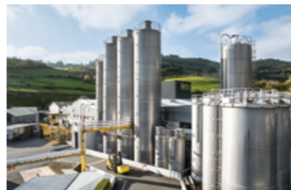
→ Modernised facilities to reduce our energy consumption. Gerflor plant, Tarare, France.
